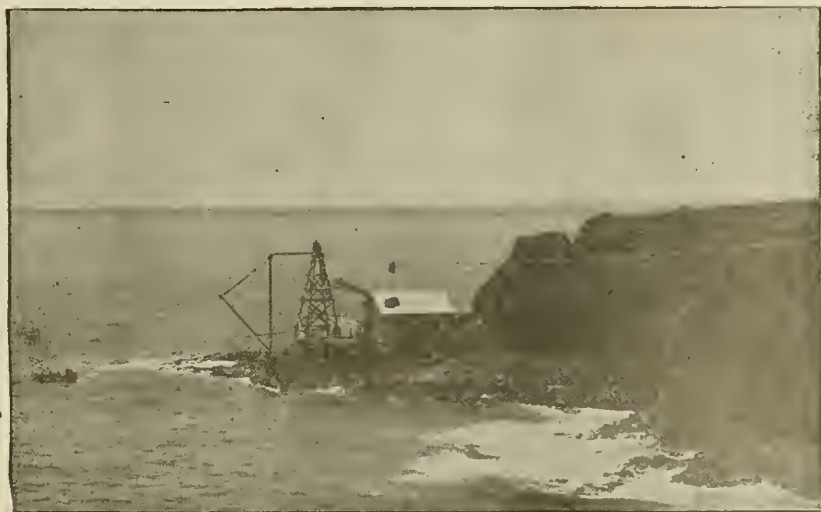
Fig. 3.—Lidgerwood Cableway, Hilo, Hawaii—Tail Tower, Warehouse Wharf and Derricks.
